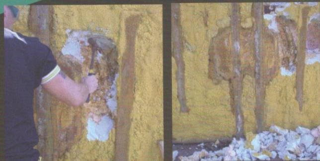
Servicing a Foamed Filled Spa
